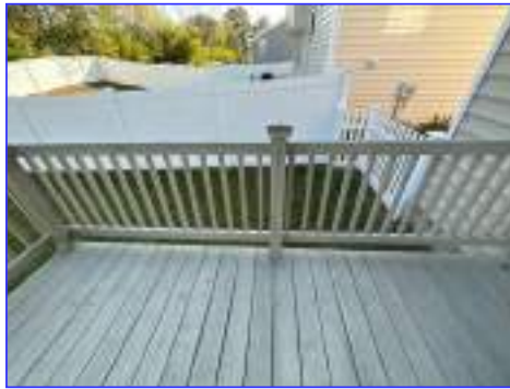
Lose guardrail
