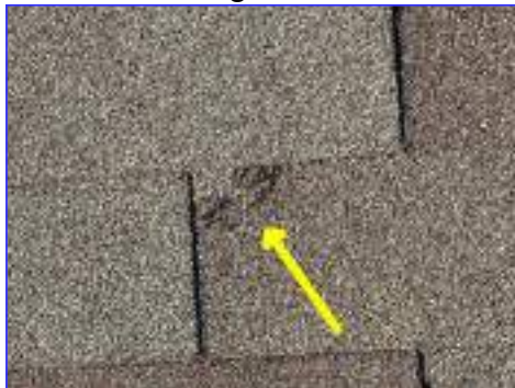
Loose/missing or damaged shingles
