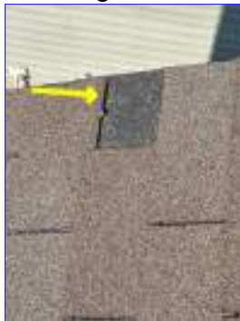
Loose/missing or damaged shingles
