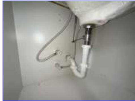
The drain assembly appears to be in satisfactory condition with no visible leaks or deficiencies.
