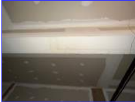
Evidence of past water penetration observed.
