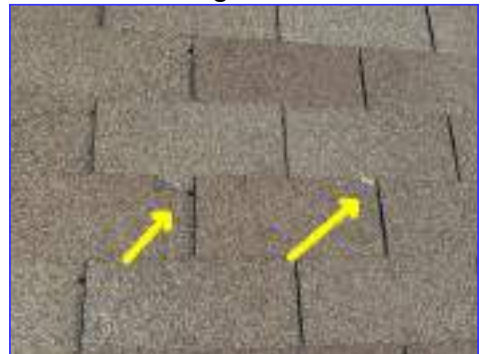
Loose/missing or damaged shingles
