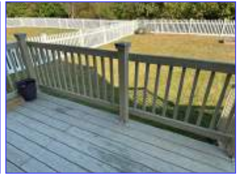
Lose guardrail
