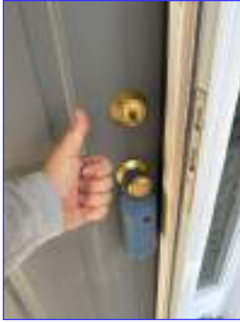
The doors are secure
