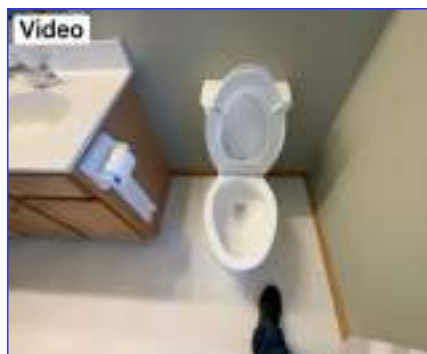
The toilet is functional with no visible leaks or deficiencies.
