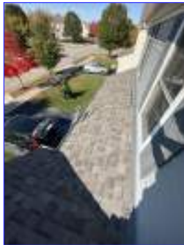
The roof shows normal wear for its age and type.
