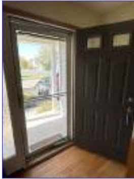
The exterior door(s) are in satisfactory condition
