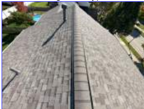
The roof shows normal wear for its age and type.
