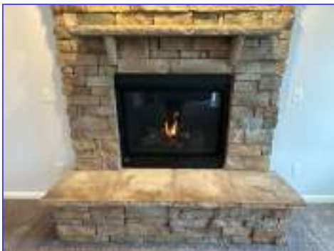
The fireplace is functional and in acceptable condition.
