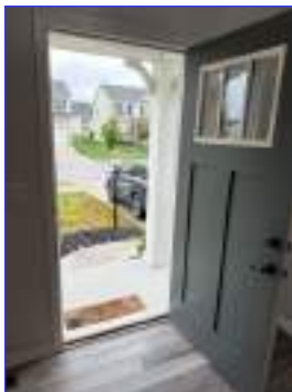
The exterior door(s) are in satisfactory condition
