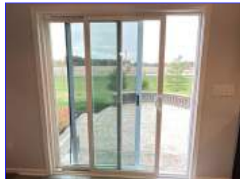
The exterior door(s) are in satisfactory condition
