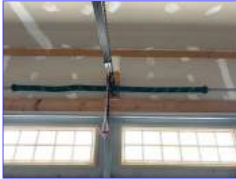
The garage door and hardware are functional.
