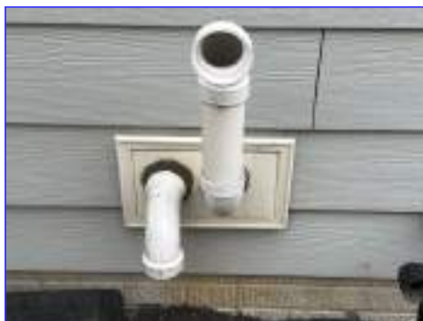
The vent pipes have no visible deficiencies.
